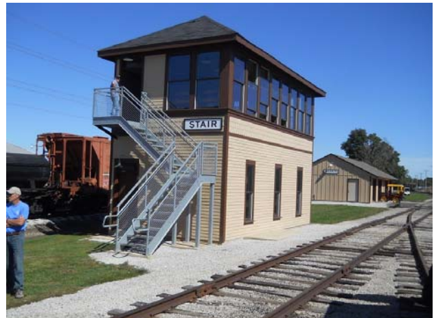
Stair Tower at the Monticello RR Museum in Illinois. It was built from Illinois Central plans and includes levers and whatnot from several demolished IC towers.
