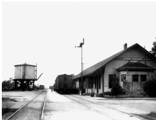
This is ACL's Perry depot where their famous Southland made its first Florida stop on its run from Chicago and the Midwest to Florida's West Coast. The Perry stop was mainly to serve the nearby winter resort at Hampton Springs. Once the Perry Cut-off was completed in 1927, this new route bypassed Jacksonville, saving 92 miles, and made the Southland the fastest train from the Midwest to Florida's West Coast. Perry was known as the Gateway to Florida's West Coast. William Money Penny photo, L.A. Bailey collection
